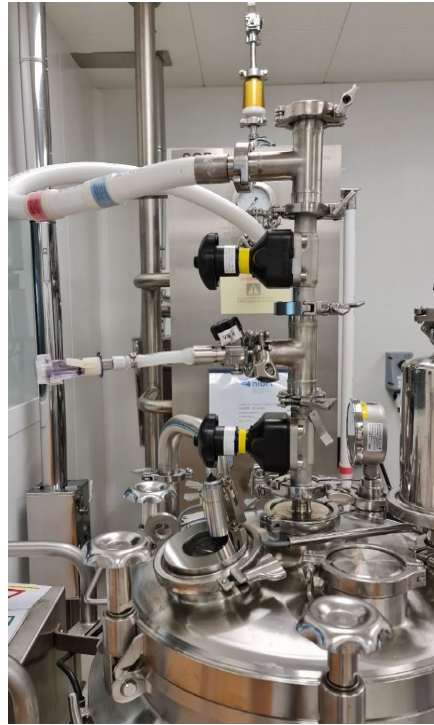
Figure 8. 3/8" ID valve connected to steaming vessel
